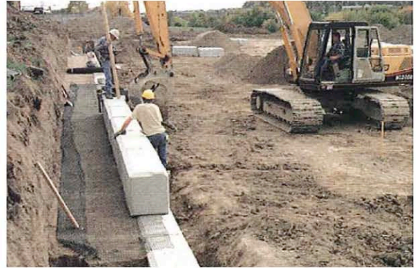
LANDMARK® blocks are a fast efficient way to install a retaining wall as each full size block cover 11.6 face sq. ft.
