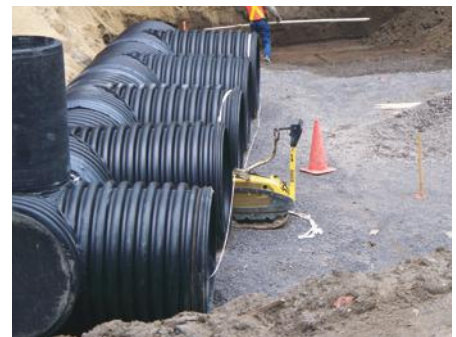
PREPARING THE SOIL FOR HDPE PIPE INSTALLATION
