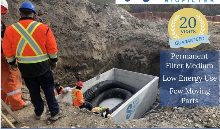
Concrete Anaerobic Digester with External or Internal Pump Tank, and Biofilter Tank
