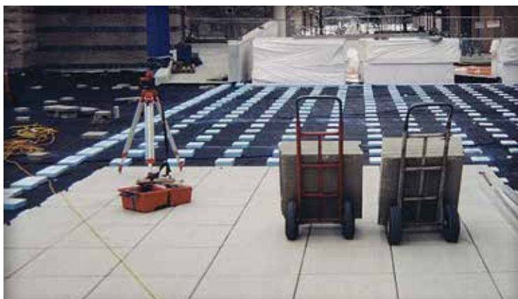
Figure 6. Foam pedestal system
