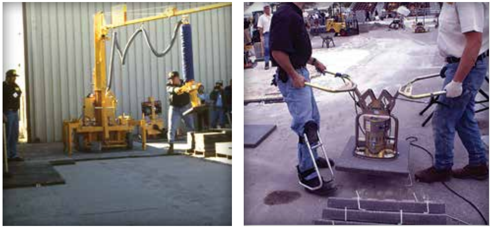
Figure 20. Vacuum assisted mechanical equipment for installing paving slabs.
